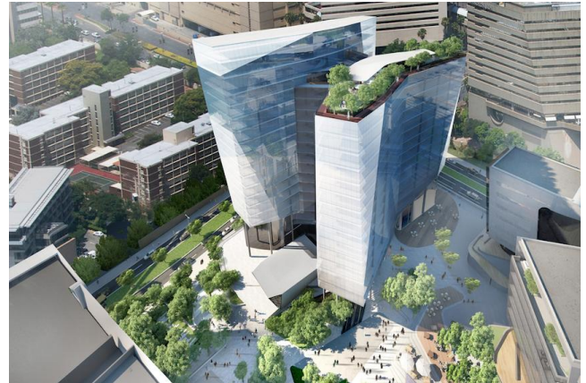
ALICE LANE PRECINCT 155 000m 2 Office Precinct with 3 buildings and super parking basement, 4 Star Green Rated
