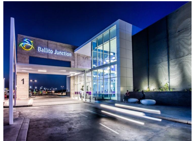
BALLITO JUNCTION 73,000m 2 Shopping Centre
